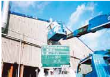
Demolition works of the former Osuga Plant No.2
