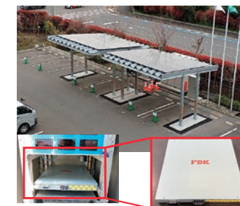
Exeo Group, Inc. Grid-free solar car port
