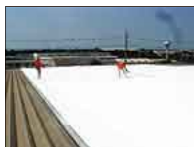
Application of heat insulating coating on the plant roof top
