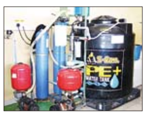
Potable water purifying system
