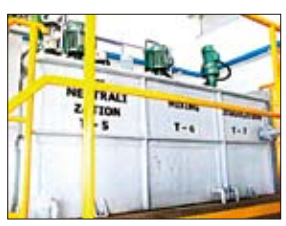
Waste water treatment facilities after an overhaul
