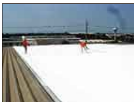
Application of heat insulating coating on the plant roof top
