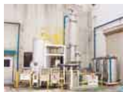
Purification system installation works
