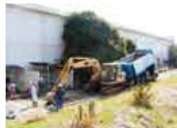
Removal by digging
