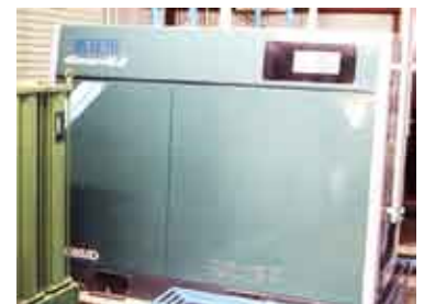
Introduction of an energy-saving type compressor (Kosai Plant)
