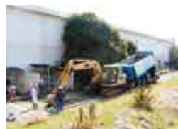
Removal by digging
