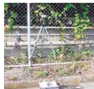
Noise and vibration measurement at the boundary of a construction site
