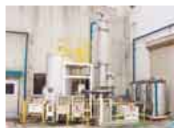
Purification system installation works
