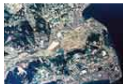
Investigation by air photos
