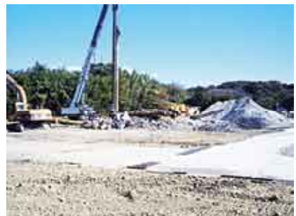
Demolishing works of the former Osuga Plant
