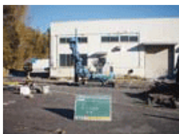
Soil Boring Investigation at Osuga Plant
