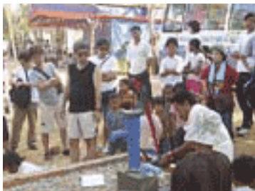
People installing a well (Cambodia)
