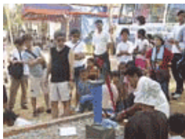
People installing a well (Cambodia)
